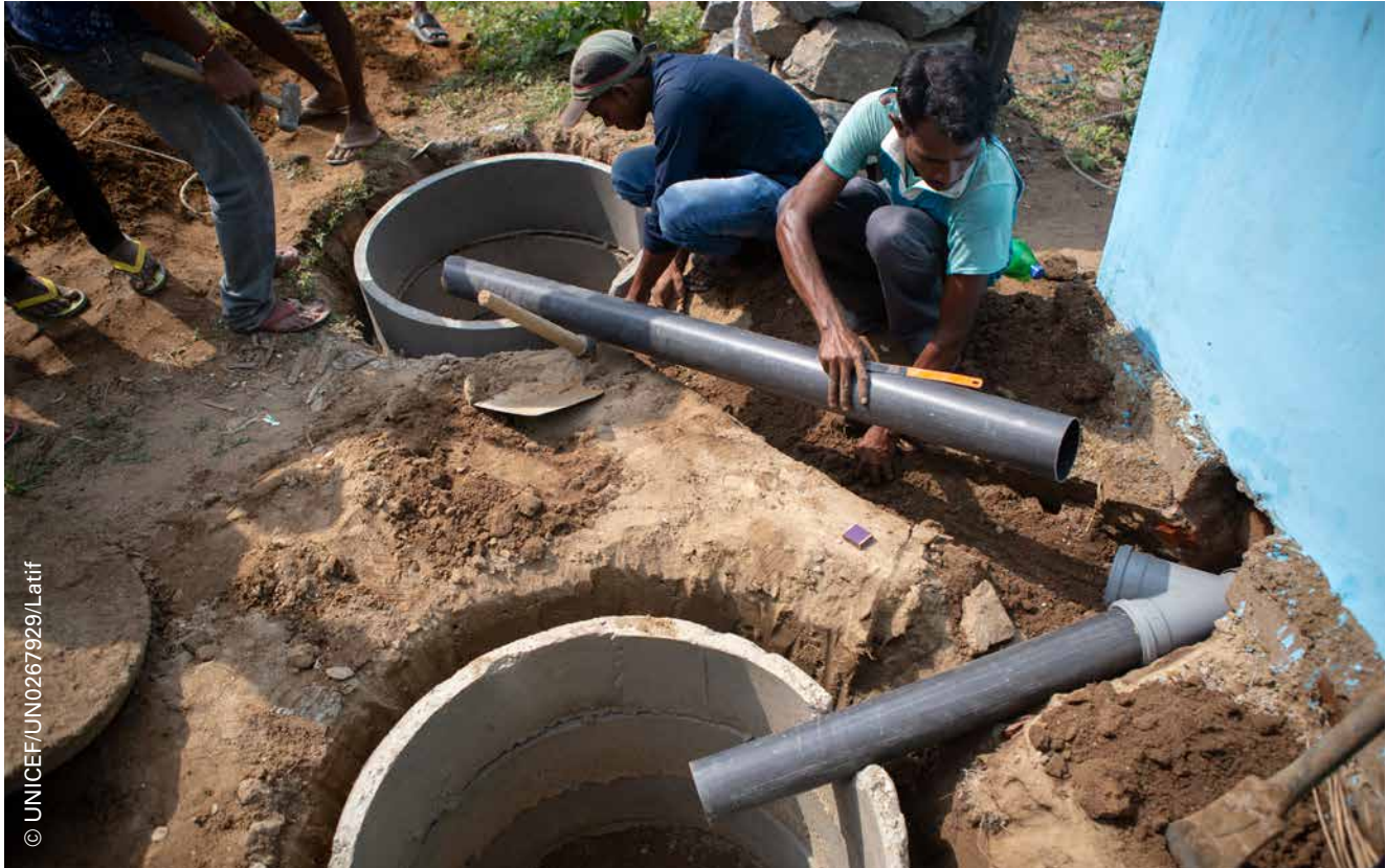
Community labourers help to construct a new double pit toilet in Nuagam village, Rayagada district, Odisha state in India.
