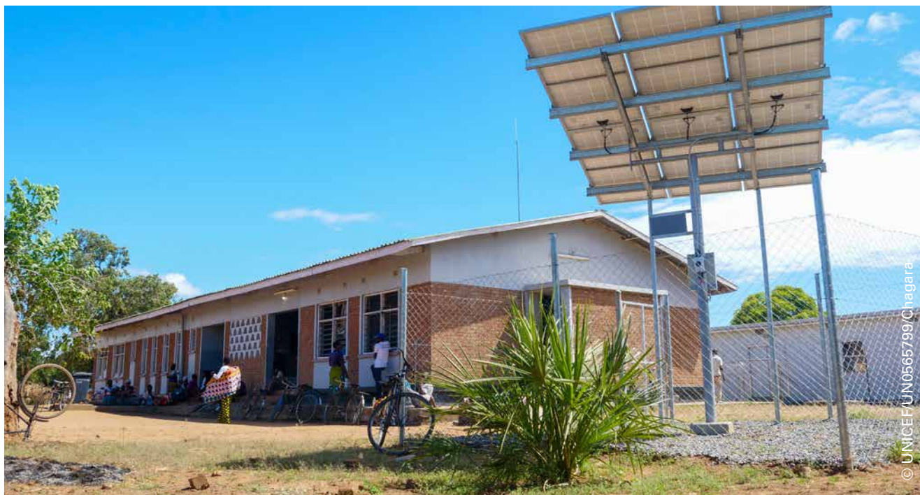
A new UNICEF-supported solar-powered water system for the Mchoka health centre in the Salima district, Malawi.
